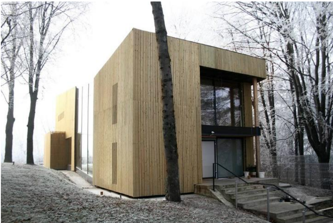
Figure 3. Passive House Che situated in Suceava County.
